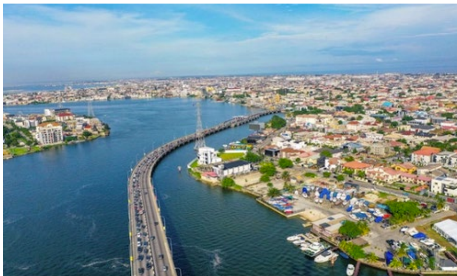
Ikoyi Bridge, Nigeria. Photo Credit: Rejoice Emmanuel, UNDP Nigeria
